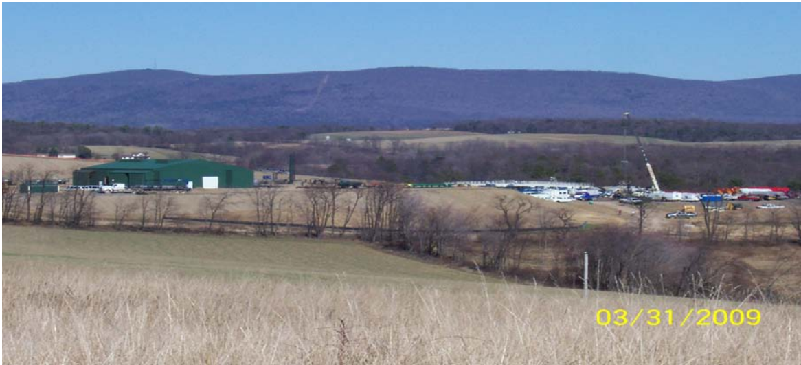
Barto Well Compressor station and well site
